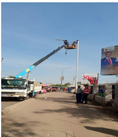
Ang'awa Avenue - Installation of solar street lighting
