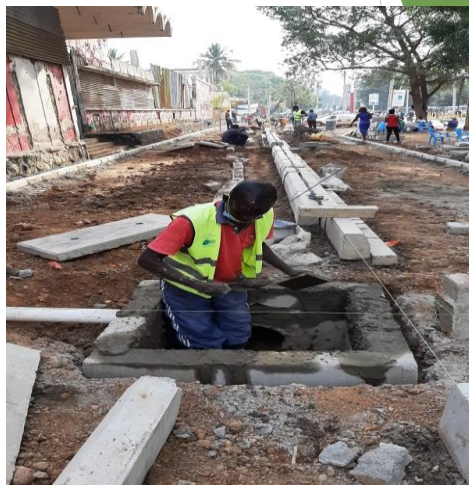
Ang'awa Avenue - Walkway, Cycle lane (notice double kerb separation) and service duct manhole works.
