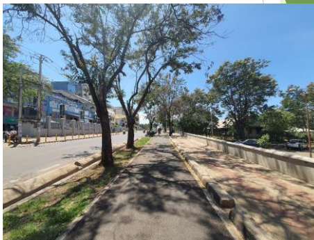
NMT section (Achieng' Oneko Road ) highlighting implemented cycle lane, landscaping (green corridor), walkway, retaining wall, bollards and drainage.
