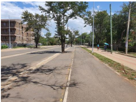
NMT section (Amolo Agar Road ) highlighting implemented side drain, parking, cycle lane, green corridor, solar street lighting and walkways.
