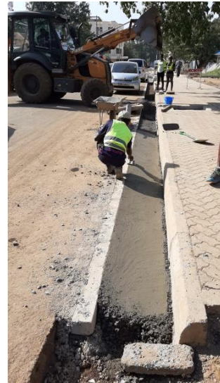
Central Police Access Road - Drainage works (Shallow side drain)
