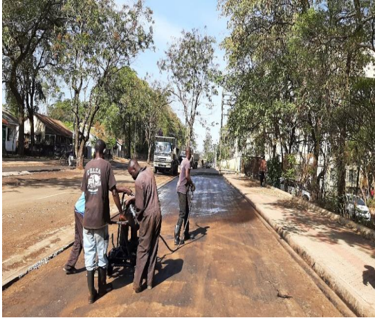
Amolo Agar Road - Priming for angular parking corridor
