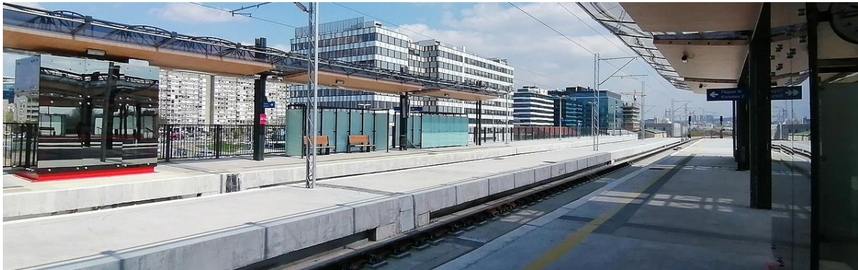
Figure 7. Novi Beograd Railway Station. Source Wikipedia.
